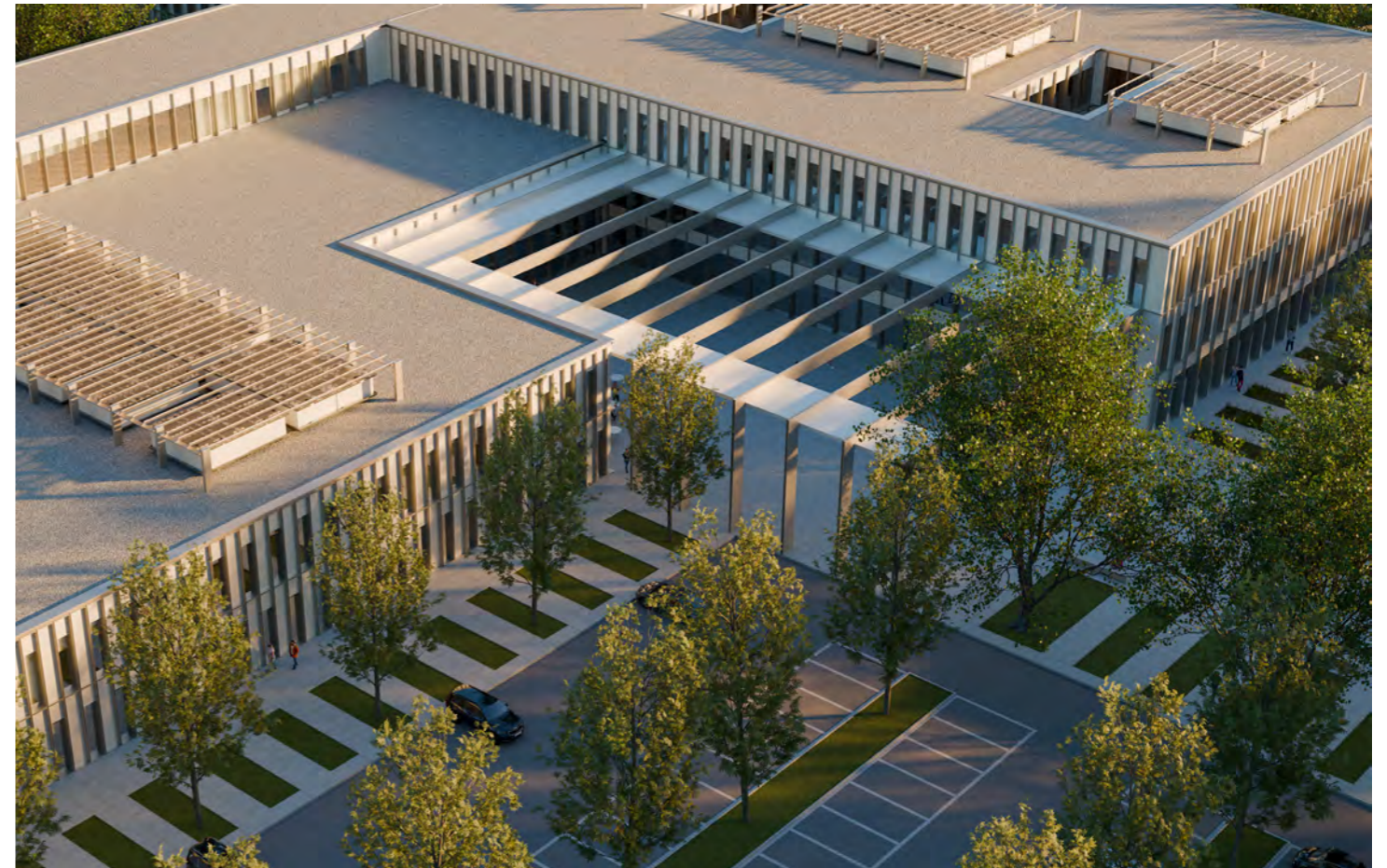
Aerial view of the main public entrance
