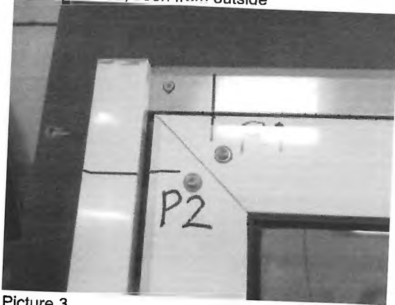
Picture 3 External corner design, casement
