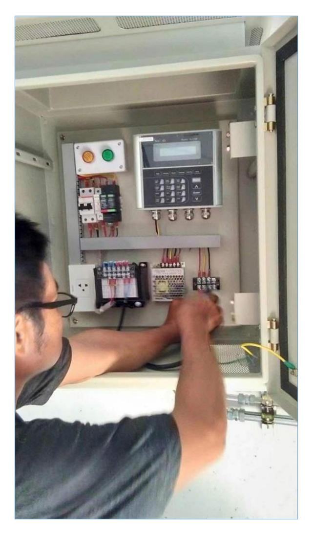
Application: Water Supply Line Model: D118 Communication: RS485 Pipe Size: DN500,DN250 Fluid: Tap Water
