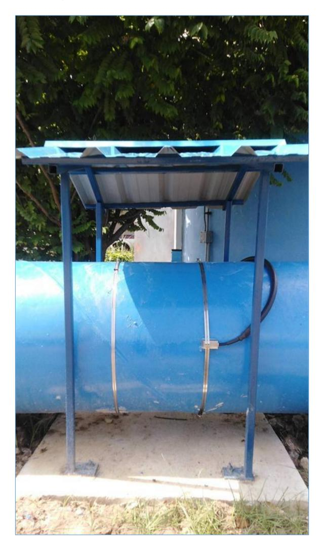
Application: Water Supply Line Model: D118 Communication: RS485 Pipe Size: DN600 Fluid: Tap Water
