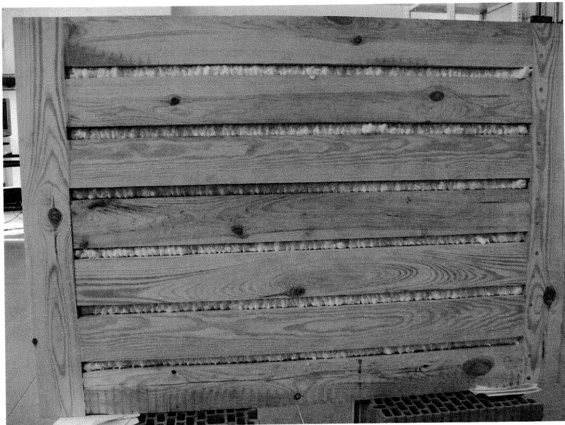
Image 1. The interstices filled with the first line of the foam
