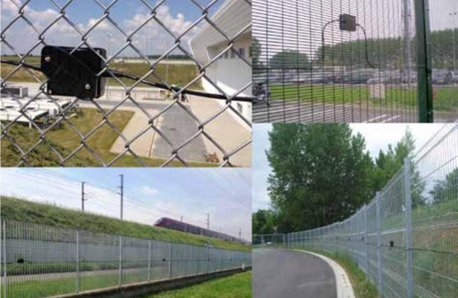
SIOUX 3.0 is our innovative IP NATIVE & PoE fence sensor system, which can protect up to 700mt and 20 zones with a single CU.
