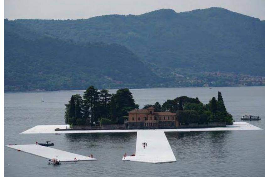
"The Floating Piers" was on display for 16 days and was visited by more than 1.2 million people. It took 4 months to construct the 3.2km-long installation, comprised of 226,000 BulDock cubes and anchored by 220 five-ton anchors. "The Floating Piers" was a modern masterpiece that created new understanding of the idea of water bodies and also affirmed that creating any form of floating structure is now possible.
