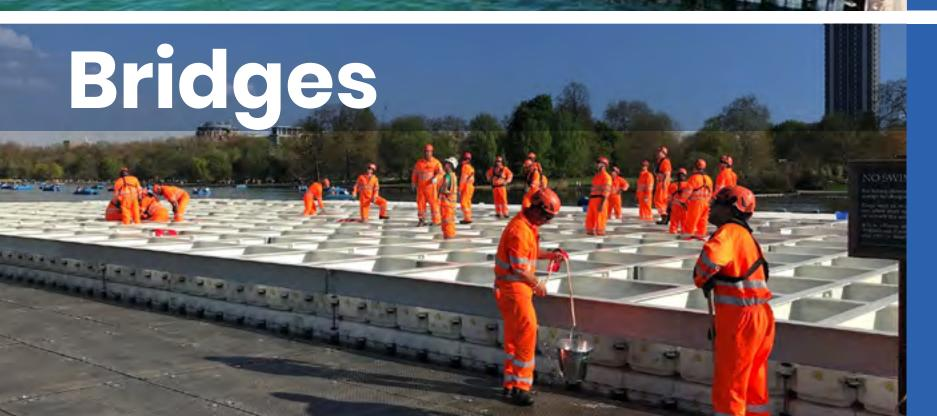
Clunky wooden and metal bridges are a thing of the past. BulDock's modular docking systems can be used to construct bridges and pathways, which are both safe (due to their anti-slippery surface) and effective (due to their high-load capacity).
