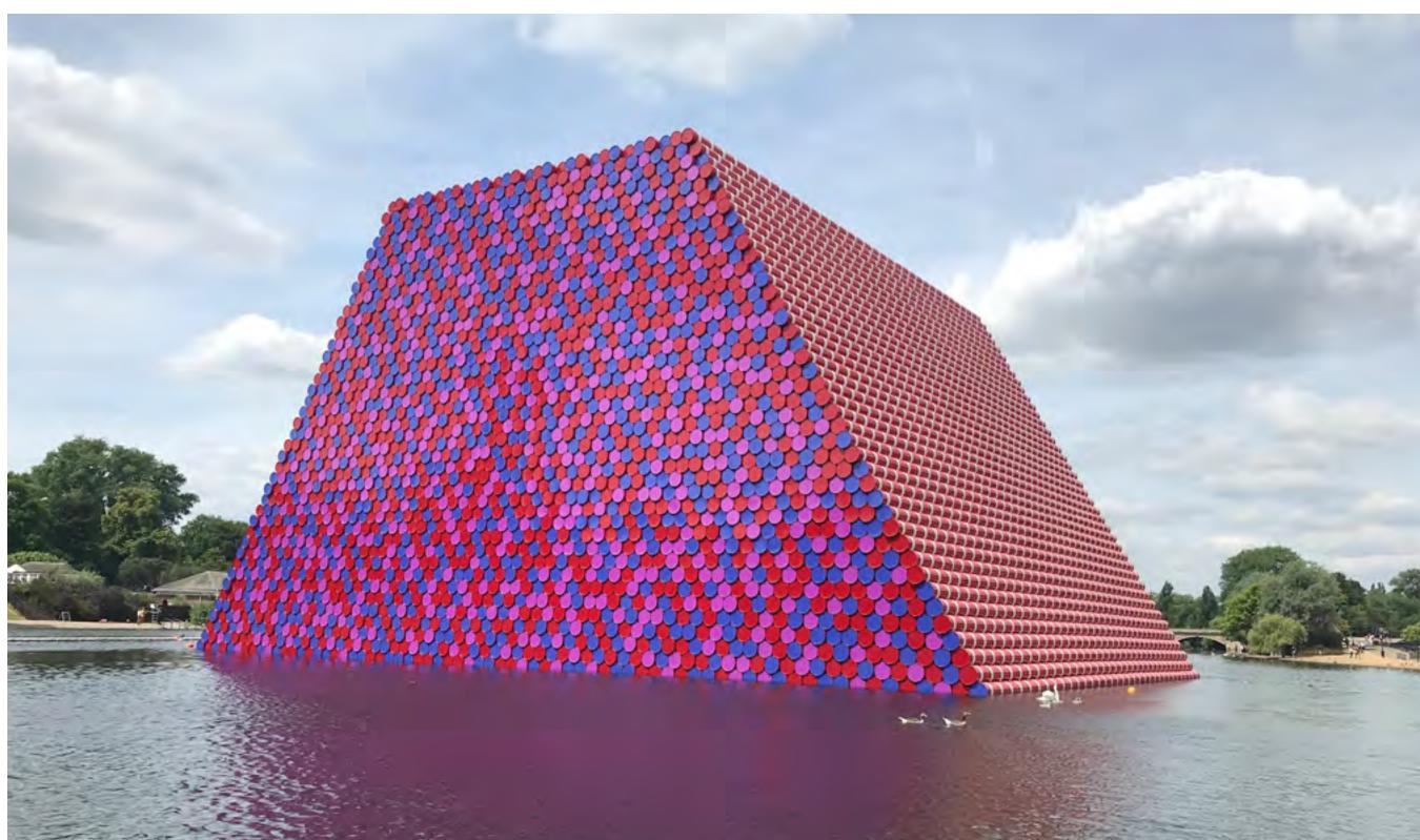
**"The London Mastaba"** (2018) at Serpentine Lake in Hyde Park was Christo's second project that BulDock was hired to execute. "The London Mastaba" was a massive 600-ton scuplture, made of 7,506 colorful barrels stacked horizontally on a BulDock floating platform. The structure was visible for 3 months and anchored to the lake's bottom with 32 sixton anchors.
