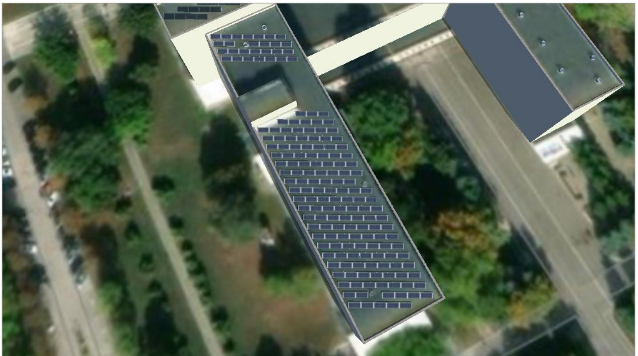
Figure: 1. Module Area - Arbitrary Building 02-Mounting Surface Northeast
