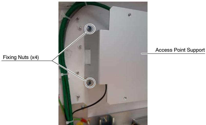
5. While holding the Access Point Support, disconnect the LAN and DC Supply Cables from the Access Point.
