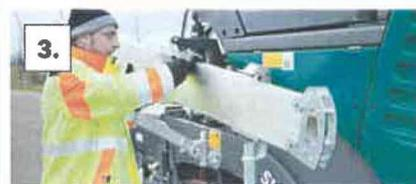
Fix the central beam in position.
