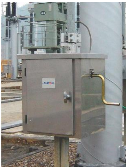
CMM Motor Operating Mechanism
