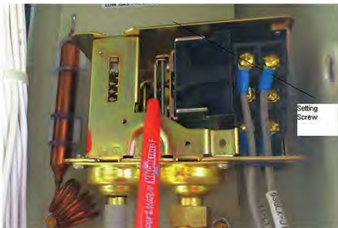
FIG. 8 CONSTRUCTION OF TEMPERATURE - COMPENSATED GAS PRESSURE SWITCH
