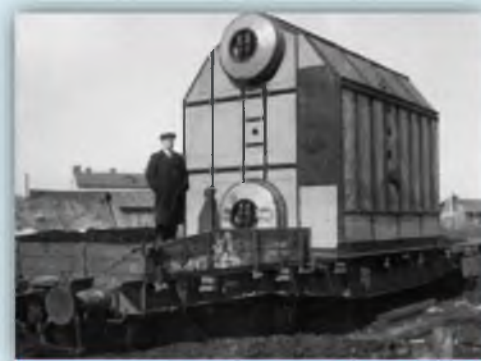
Experimental Steam boiler of CKTI TK-3-13 system
