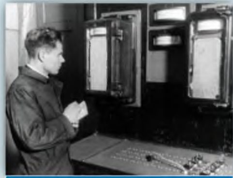
Senior Engineer of CKTI A. A. Kanaev is taking readings of recorders installed on the experimental binary plant, GES No. 4, 1937
