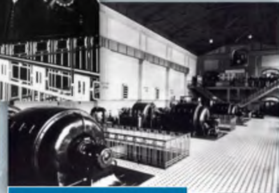
Generator hall interior, 1907
