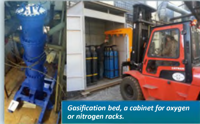
Gasification bed, a cabinet for oxygen or nitrogen racks.
