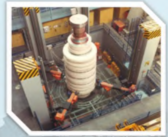
Welding of root parts of rotor welds
