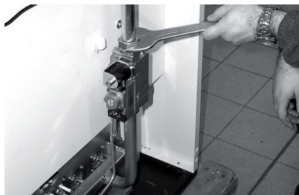
fig. 9 - Undo the gas valve nut
