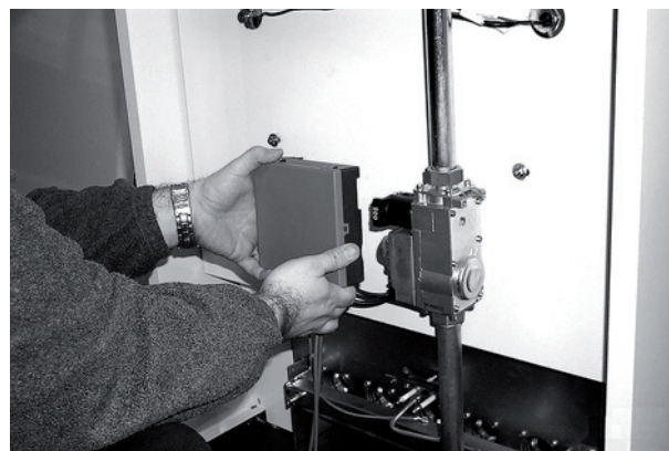
fig. 8 - Remove the control unit
