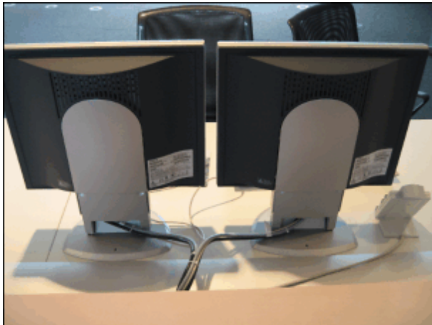
Fig. 79: Laying the monitor cables
