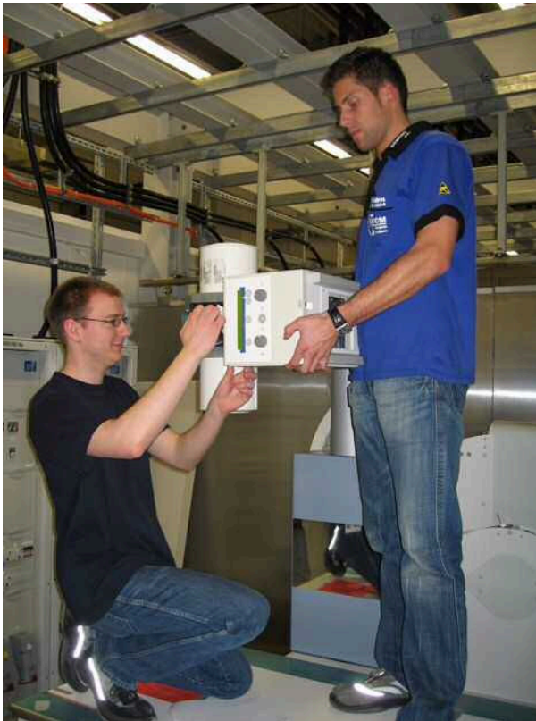
Fig. 39: Installing the collimator
