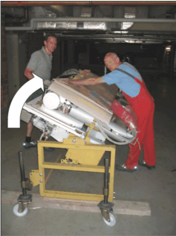
Fig. 13: Pivoting the unit support
