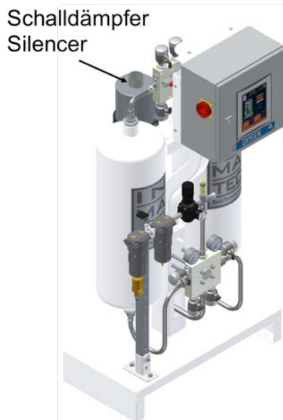
Fig. 2: Silencer connection
