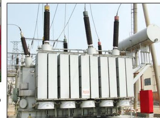
在河南焦作运行的220kV油浸式电力变压器 220kV Oil-immersed Power Transformer isoperating in Jiaozuo, Henan province
