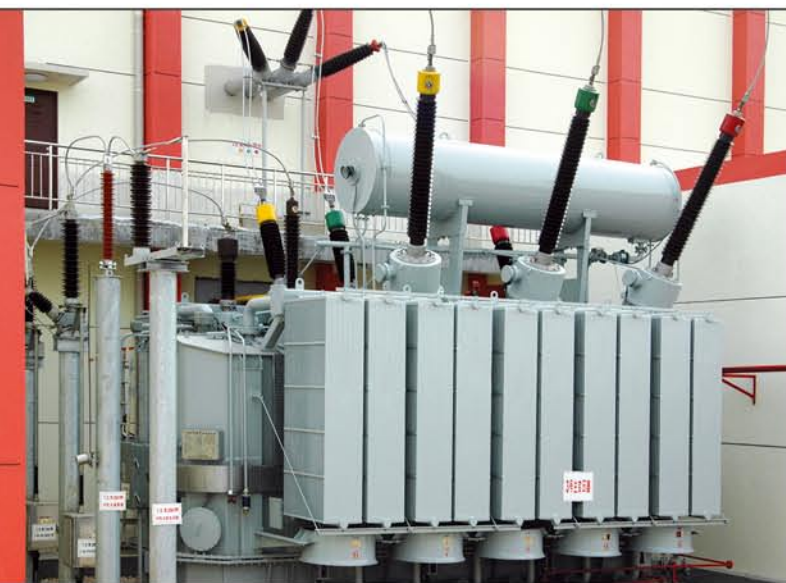
在国家电网运行的220kV油浸式电力变压器 220kV Oil-immersed Power Transformer is operating in National electrical network
