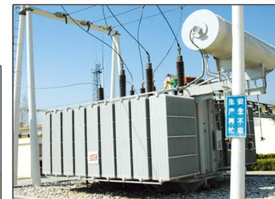
运行中的110kV油浸式电力变压器 110kV Oil-immersed Power Transformer is Operating in State Grid
