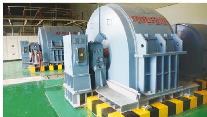
工频发电机组 (30000KVA 50HE/60HZ 7500KVA 200HZ) Power frequency generating set (30000KVA 50HE/60HZ 7500KVA 200HZ)
