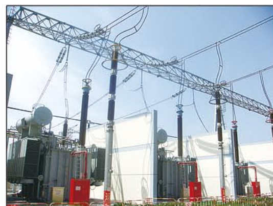
在山东郛城挂网的500kV油浸式电力变压器 500kV Oil-immersed trandformer is operating in Yuncheng, shandong Province
