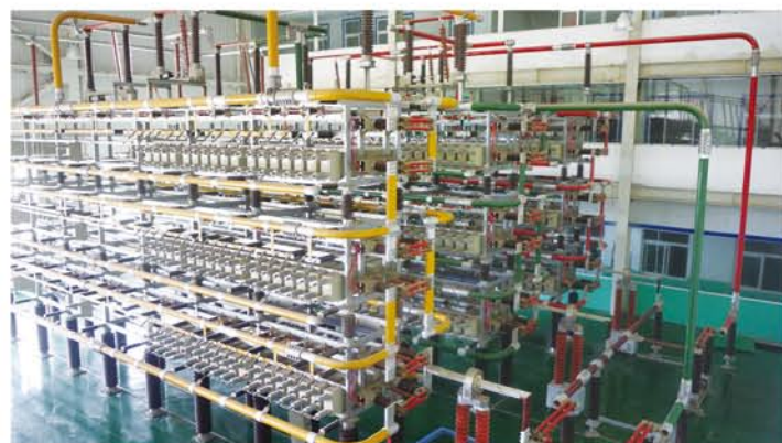
9.388800K Var补偿电容器 388800K Var compensating capacitor
