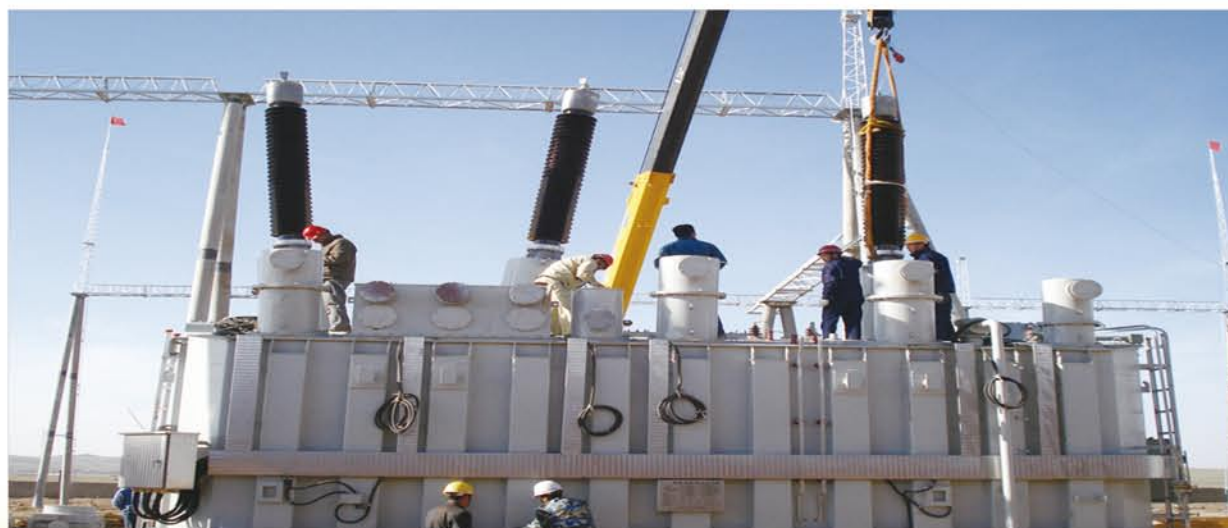
达驰公司服务人员在内蒙古中旗风力发电厂安装220kV级180MVA变压器 .The service personnel of Dachi company in Inner Mongolia Zhongqi wind power plant are installing the class 220kV 180MVA transformer.
