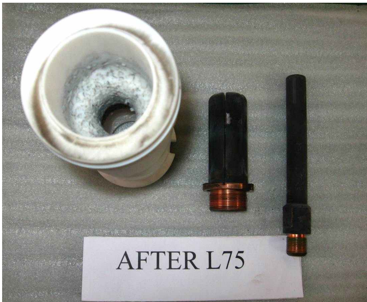
Photo. HP08 : Contact after short line fault (L75)
