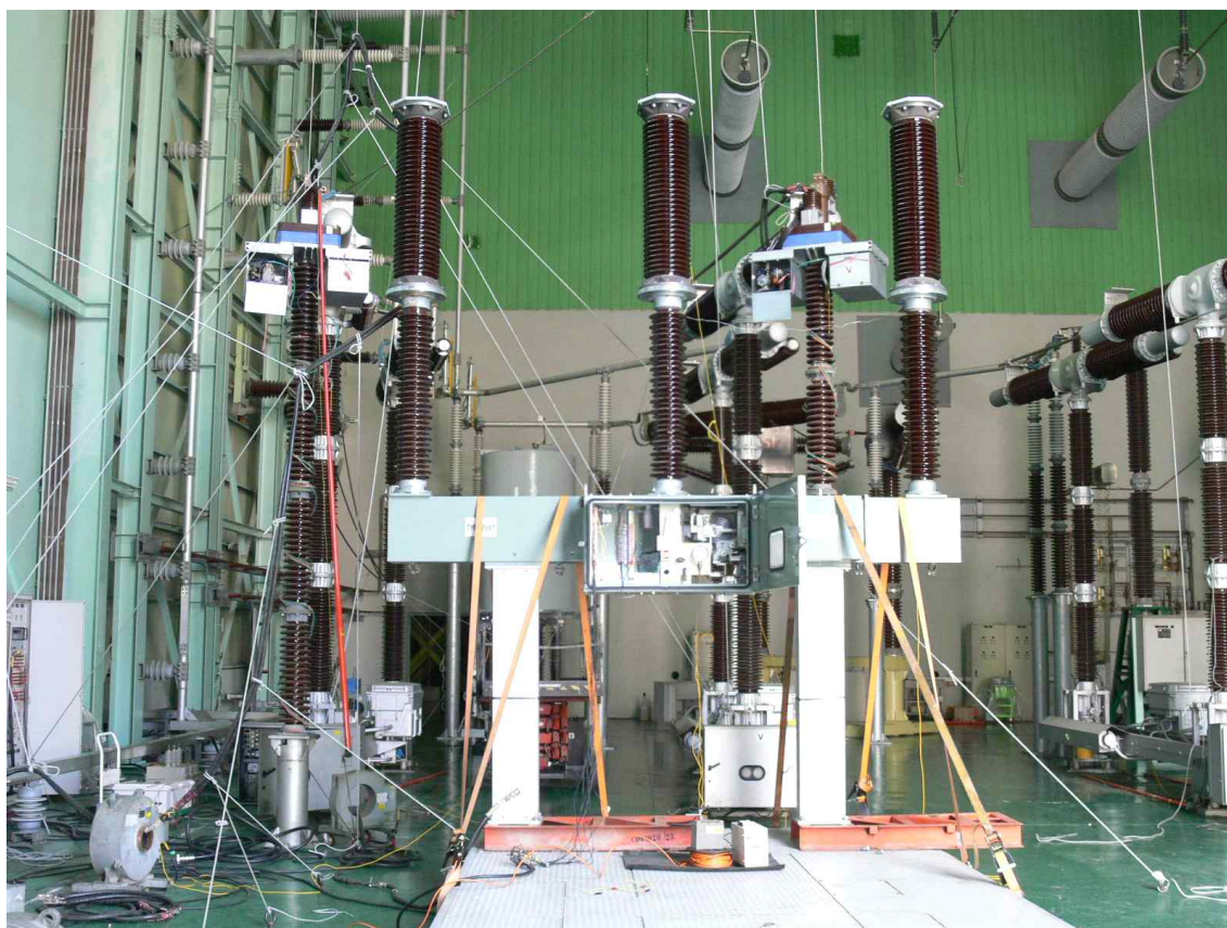
Photo. HP01 : After basic short circuit tests(T100)
