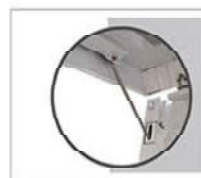
Iron hook support rod for panel support
