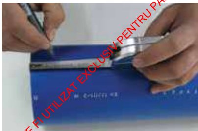
Measure and mark the pipe
