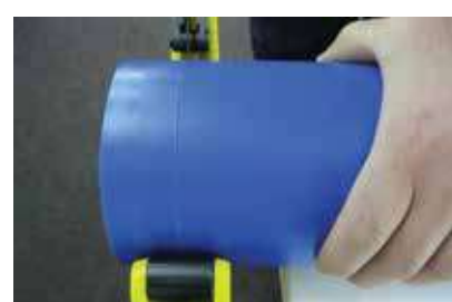
With light circular movement, cut the outside PP layer
