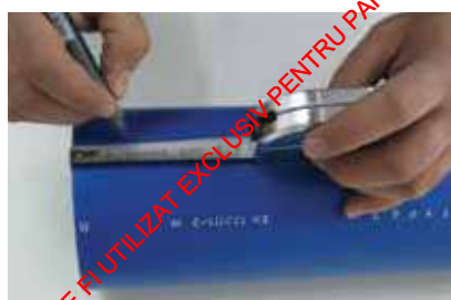
Measure and mark the pipe
