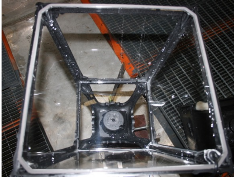
Photograph No. 57 Components plate after removing the cover.
