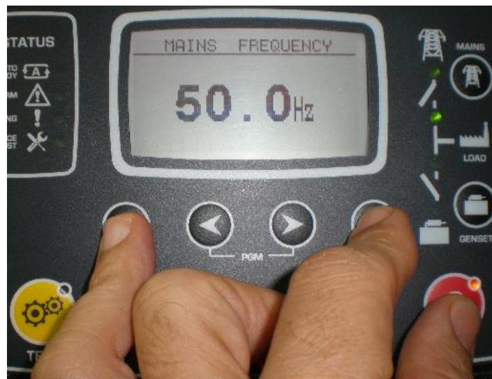
Hold pressed STOP, LAMP TEST and ALARM MUTE
