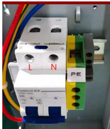
Figure2-4 Single phase-three-wire connection
