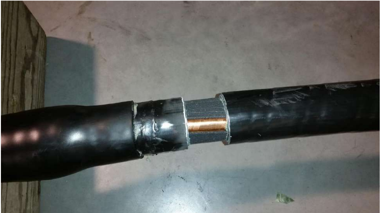
Cable oversheath removed according clause 9.3 of IEC 61442.
