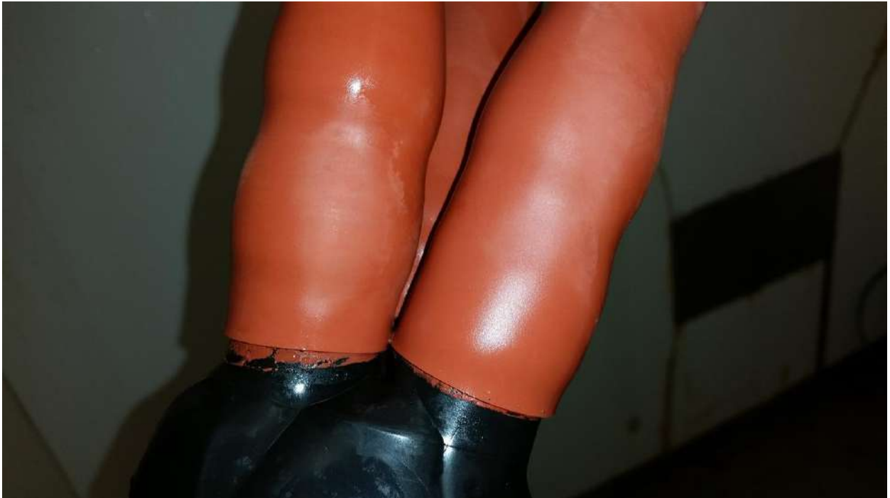
Detail indoor termination after test
