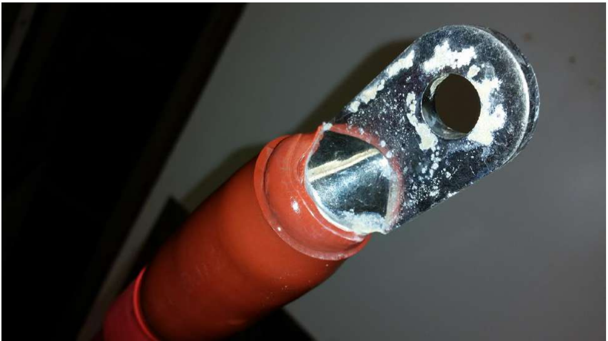
Detail indoor termination after test
