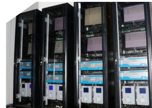
Installation of online exhaust gas monitoring equipment
