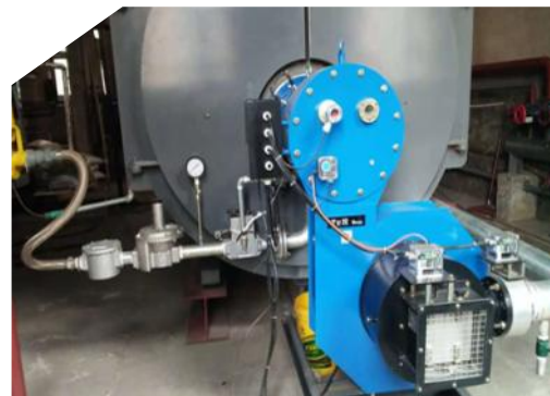
Gas Fired Boiler-the first to use low-nitrogen burners, ultra-low exhaust gas emissions
