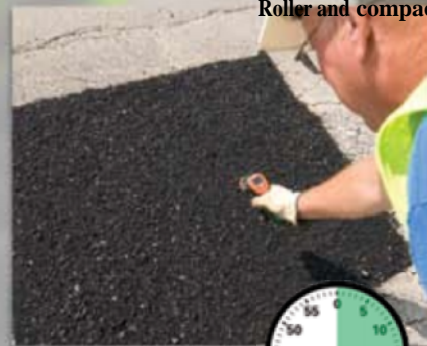
Temperature check and apply ASP Sealer
